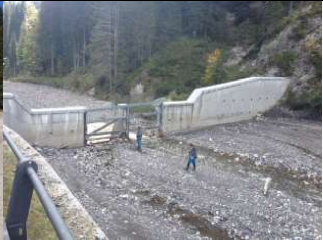
Photo 6. Individual Inspection Test 2 (Day 1)
