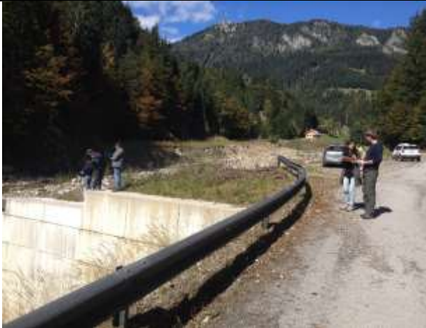
Photo 5. Individual Inspection Test 2 (Day 1)
