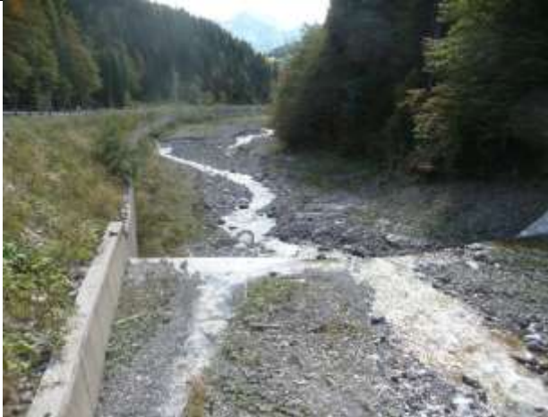
Photo 3. Individual inspection Test 1 (Day 1)
