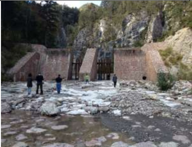
Photo 7. Individual inspection Test 3 (Day 1)
