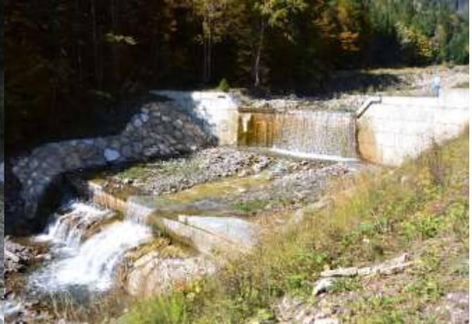
Photo 4. Individual inspection Test 1 (Day 1)
