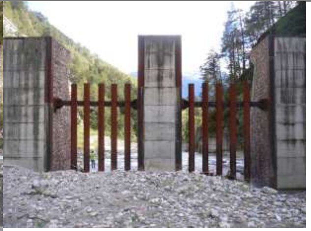
Photo 8. Individual inspection Test 3 (Day 1)
