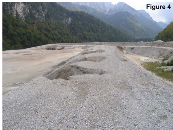
Figure 3. Erosion channel cut through the embankment of a tailings pond.
