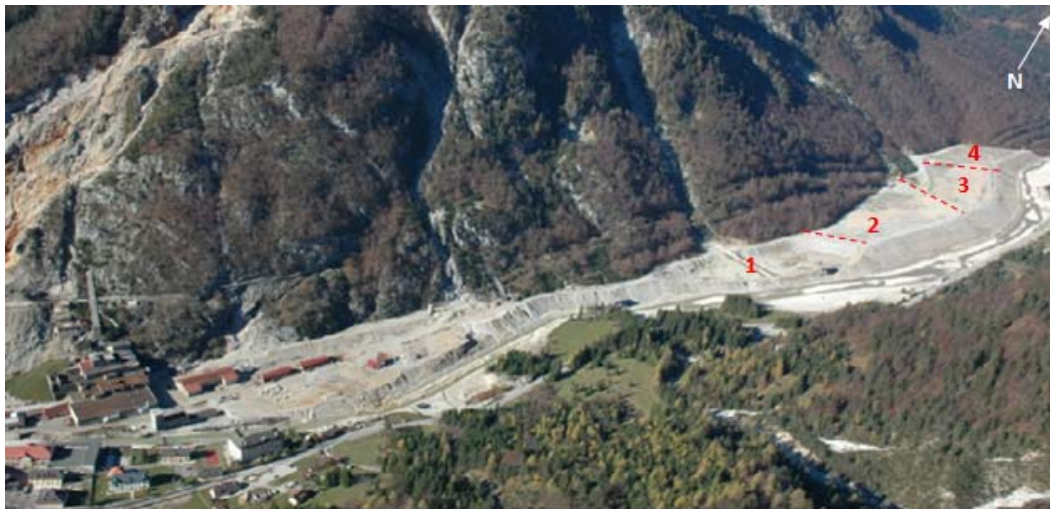
Figure 1. Aerial view of the old flotation plant area and the tailings ponds.
