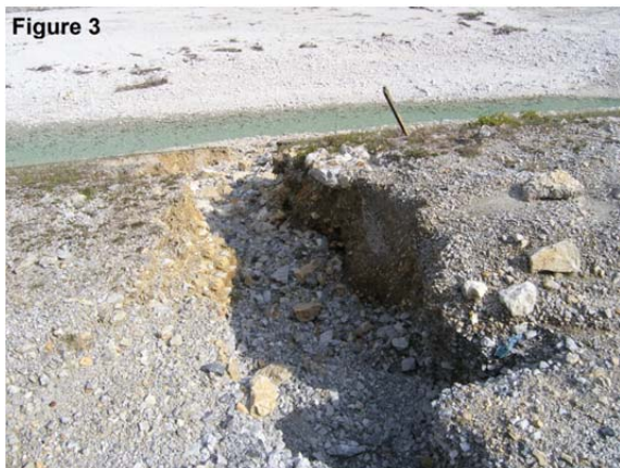
Figure 3. Erosion channel cut through the embankment of a tailings pond.
