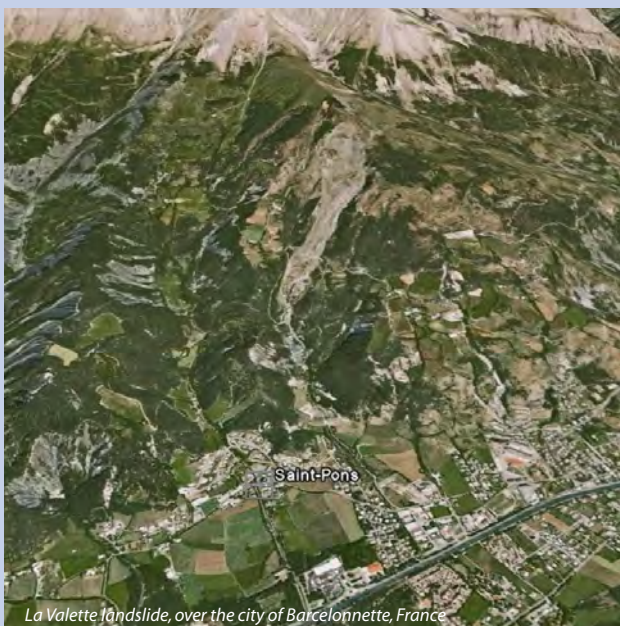
La Valette landslide, over the city of Barcelonnette, France
