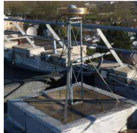
Steel mast (Toulouse)
